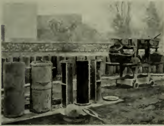
FIG. 1. MOULDS AND MANDREL.
